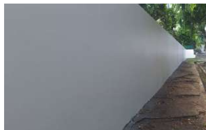
After Rectification Works
