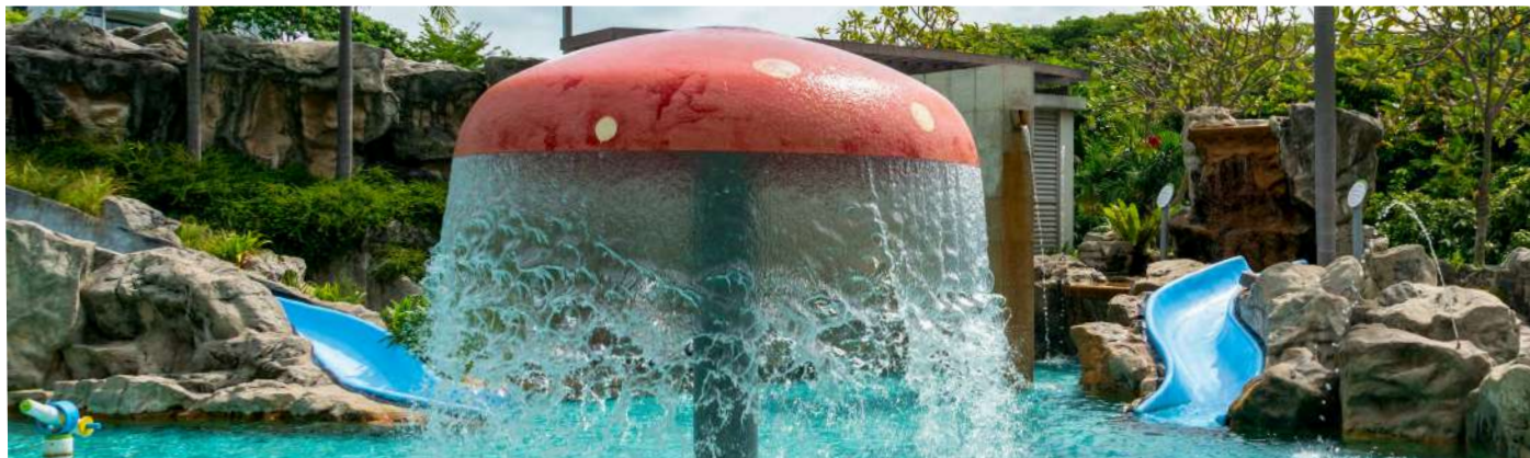
Repaired and repainted Fun Pool slides
